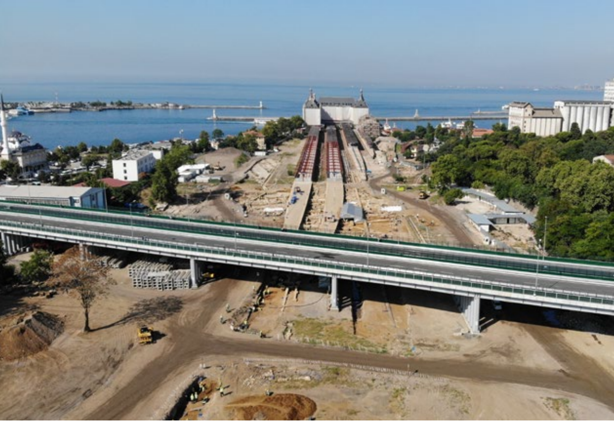
Haydarpaşa Railway Station Overpass Bridge
